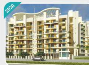
SAI DHAM RESIDENCY Adjacent BHS, Civil Lines, Prayagraj
